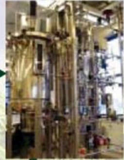
Archer Daniels Midland is constructing a fermentation plant in Clinton, Iowa.
